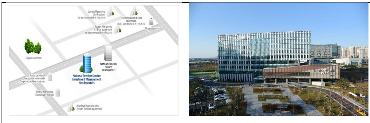
<NPS Investment Management building>
